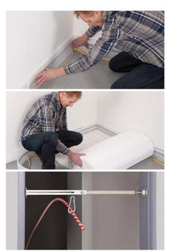
Efficient unwinding of the Pe-Xcellent and the aluminium composite hook-and-loop piping are made possible with the intelligent pipe unwinding aid.
